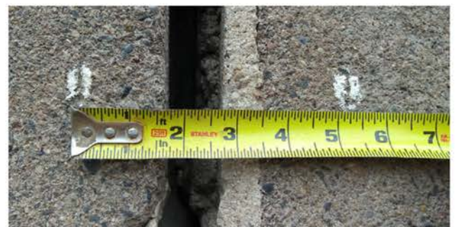
The width of the crack after rotation had occurred grew approximately 3/8" , a measurement consistent with the Veva III Tilt Monitor's reading of 0.04^\circ .
